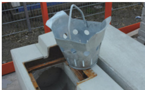
Installed sump unit
